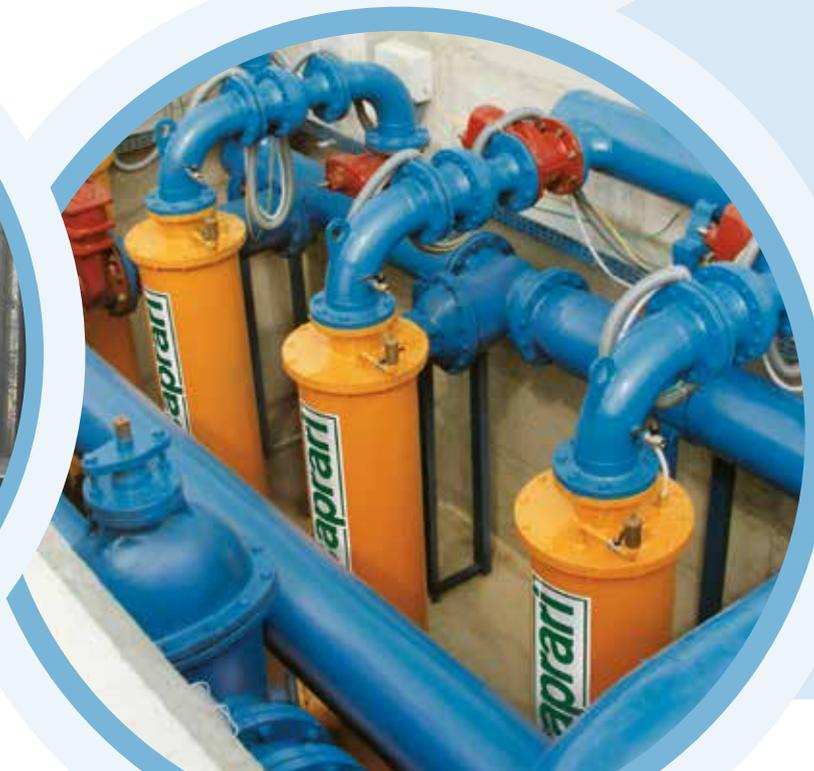
The containers may be made of galvanised steel or stainless steel. They can also be equipped with a variety of accessories, such as devices for protection against operating in a dry condition, or sensors for max./min. pressure, etc.
